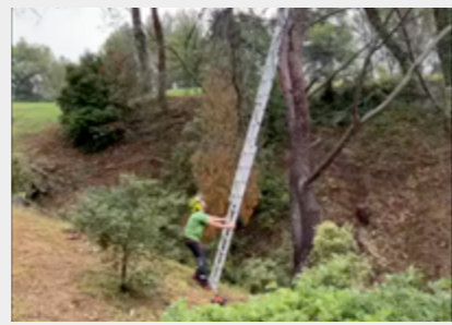
Pruning work as part of brush clearing operations on Boulevard du Roy René.
