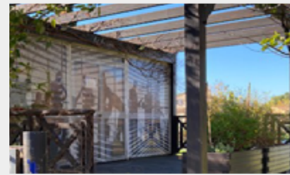
Moving the Kiosque structure to the Canal Parking to create a storage area.
