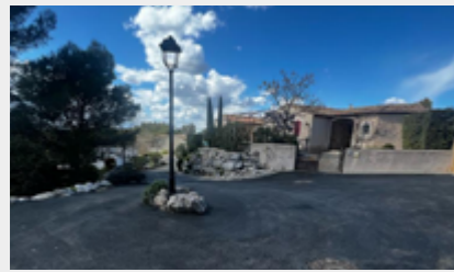
Renovation of asphalt of the street at La Citadelle 2.
