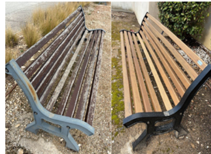
Refurbishment of benches (paintwork and seats)
