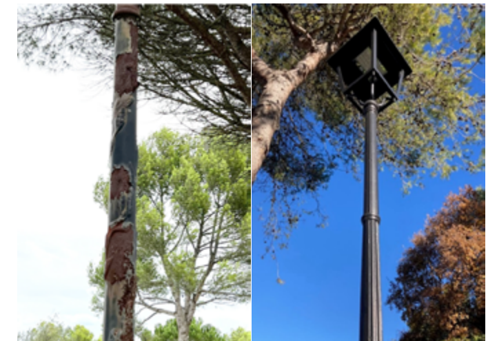
Refurbishment and repainting of lampposts
