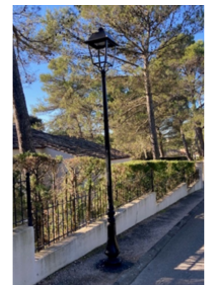
Replacement of a streetlight rue des Vallons (following an accident)
