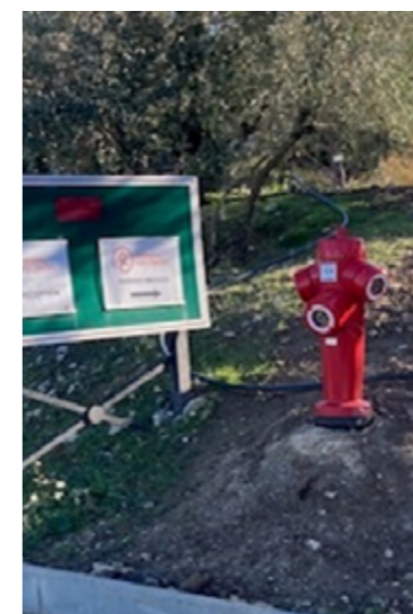
Replacement of a fire hydrant
