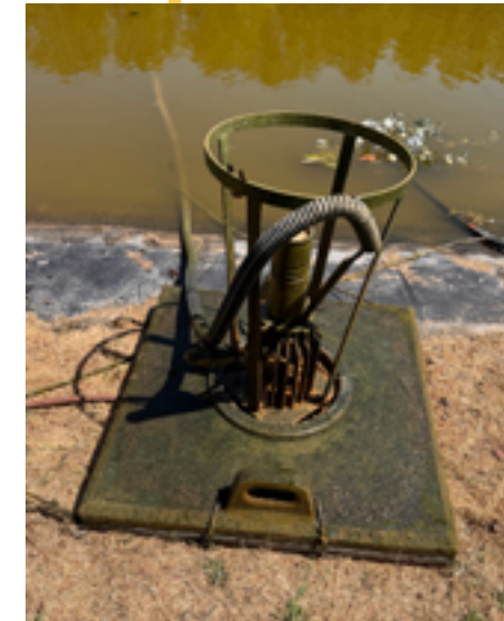
Repair of the water jet on hole 10
