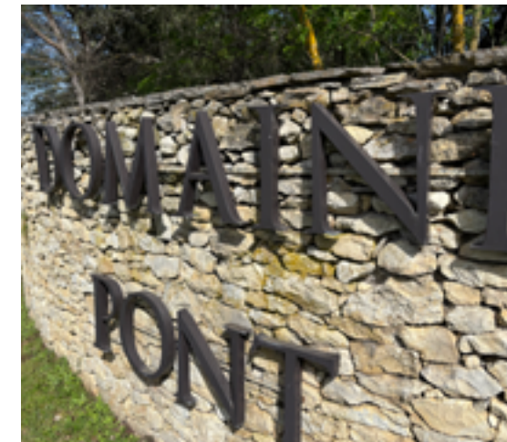
Cleaning and anti-fungal treatment of the outside wall (roundabout) and the wall at the bend in rue de Vernègues (at the bottom of hole no. 1)
