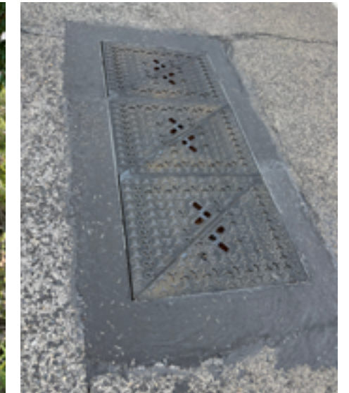
Consolidation of manhole covers
