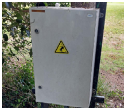
Repairs following electrical failures (Rue de Vernègues, Micocouliers)
