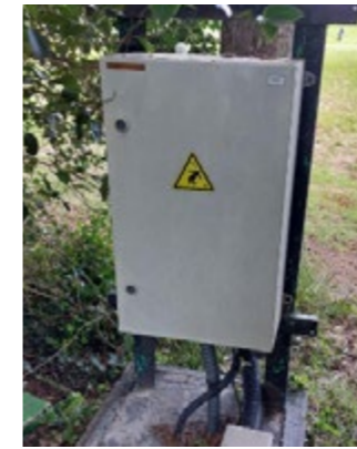
Replacement of electrical cabinet (cables damaged by rodents)
