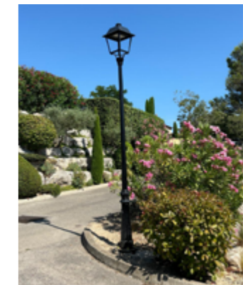
Installation of a lamppost at Citadelle 2
