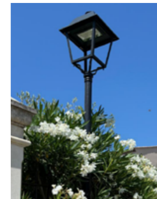
Securing damaged lighting at the guardhouse.
